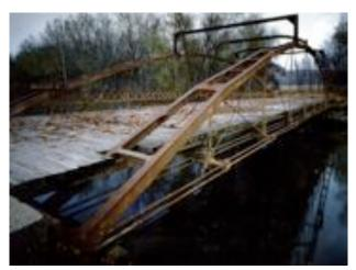
It took a practical American fellow, Squire Whipple b 1804, d 1888 to design a bowstring iron truss bridge in 1840. An arch in compression needs a huge base to constrain the outward thrust of arch forces. Whipple put a bowstring between the bases. Whipple's bowstring, a base in tension, removed the need for massive piers to constrain the arch from spreading out. Arch bridges could now be prefabricated and carry load without counting on massive end piers to prevent the arch from collapsing.
